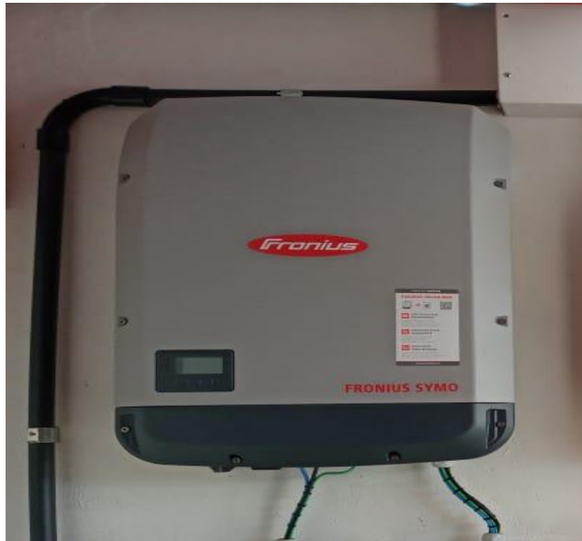
Figura 6 – Inversor FRONIUS
